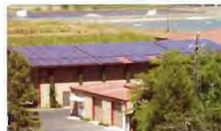
The Ballentine Vineyards 87 kW solar system will pay for itself in just six years.
