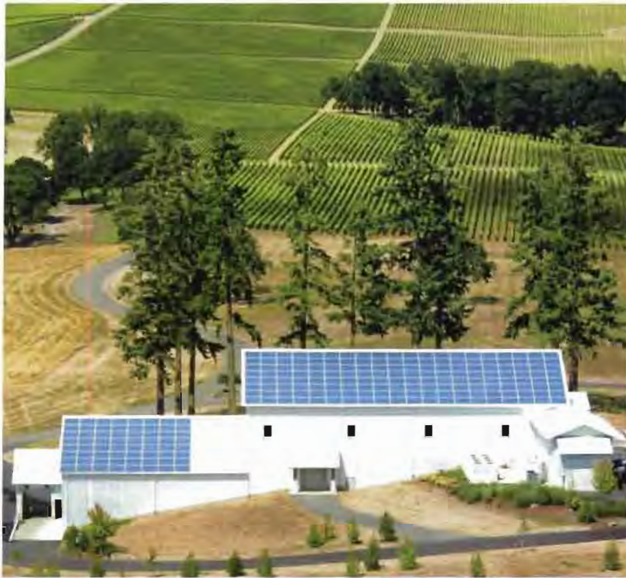
Stoller Vineyards (Dayton, OR) installed a 244-panel PV system as part of the LEED-certified winery built in 2006.
