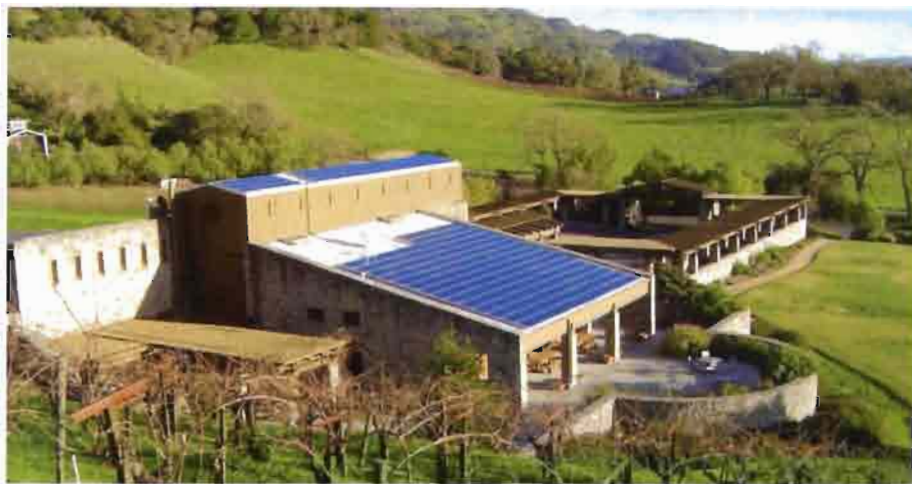
33.3 KW solar system at Robert Sinskey Vineyards, Napa. Panels are west-facing, with the larger array on a 20° slope and the smaller on a 10° slope. With five inverters, real yield of the panels averages about 28 KW. Phase II — a second PV system estimated at 35 KW, will be installed on the parking lot trellis structure in 2005. Photo courtesy REC Solar
