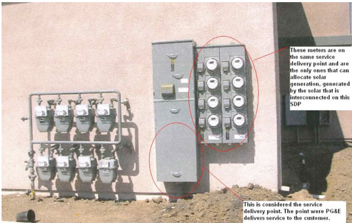
Figure 1: PG&E's diagram of the only circumstance under which a customer can participate in VNM.
